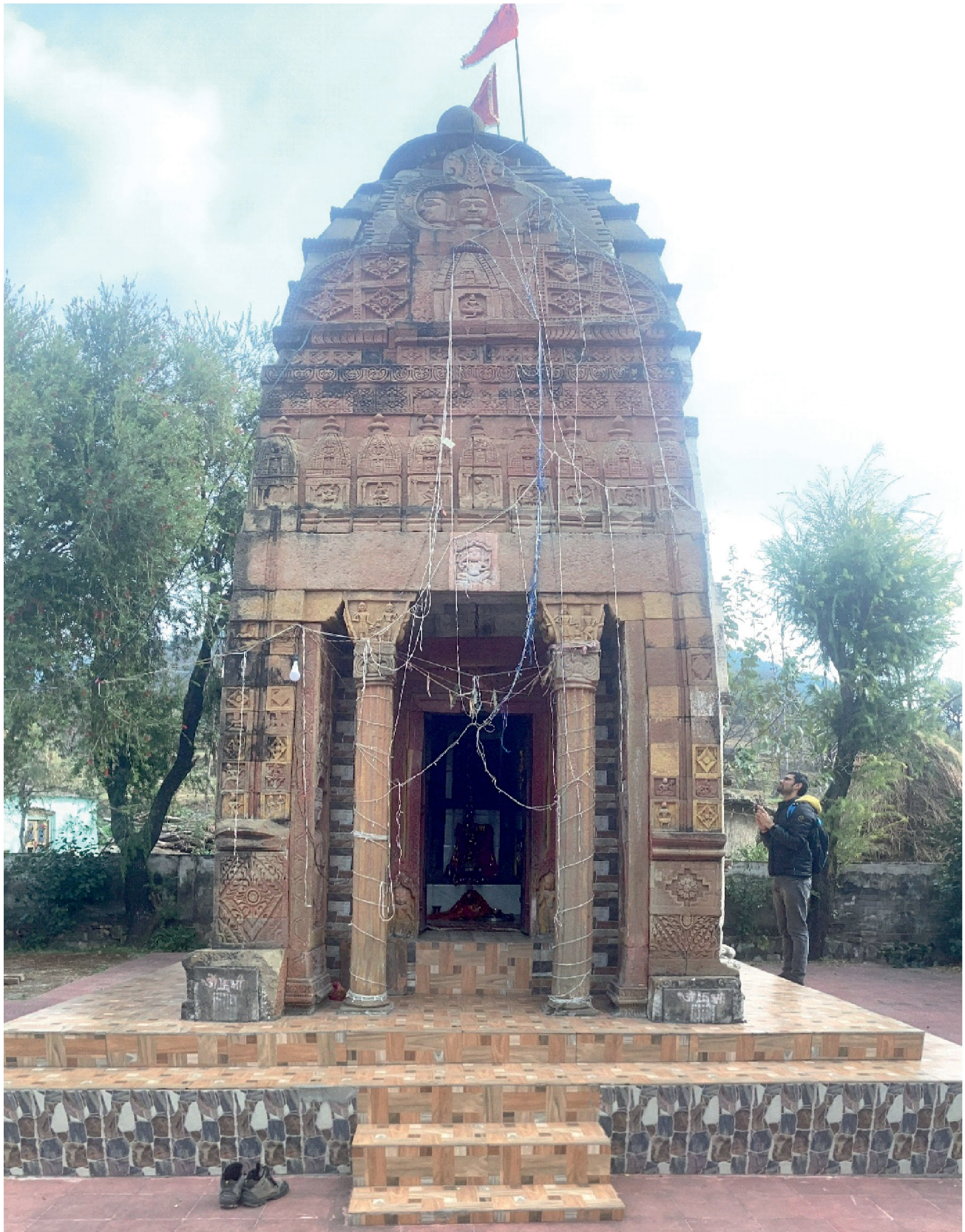
Fig. 6: Front façade of Jalandhara Devi Temple (west side)
